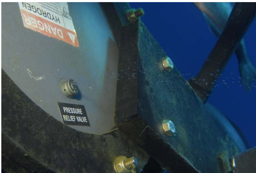
Figure 1. A significant amount of H 2 bubbles blowing from the battery pressure relief valve.
